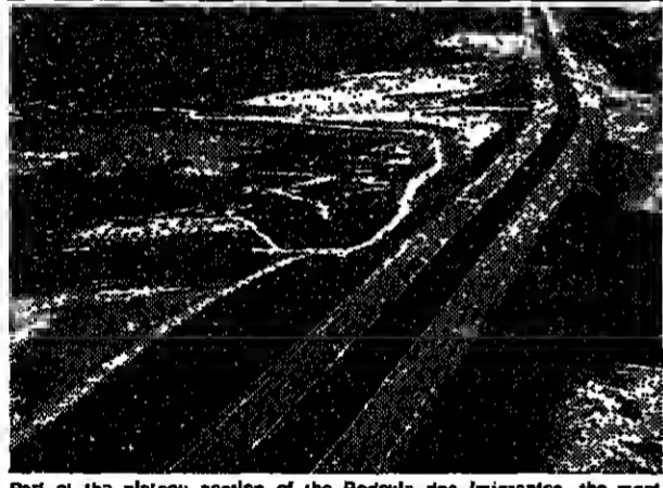
Part of the plateau section of the Rodovia dos Imigrantes, the most modern motorway in Brazil, linking its leading industrial centre with its largest port.
